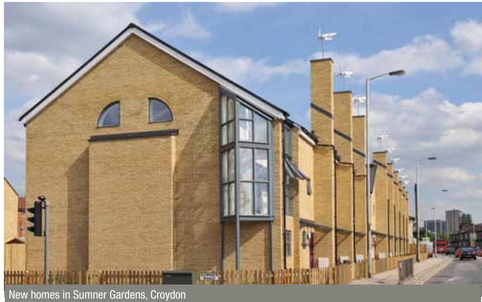
New homes in Sumner Gardens, Croydon
