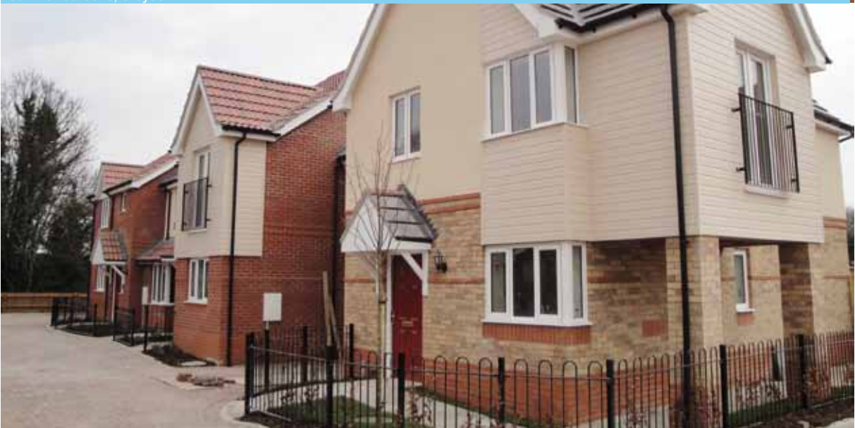
New build at North Kesteven
