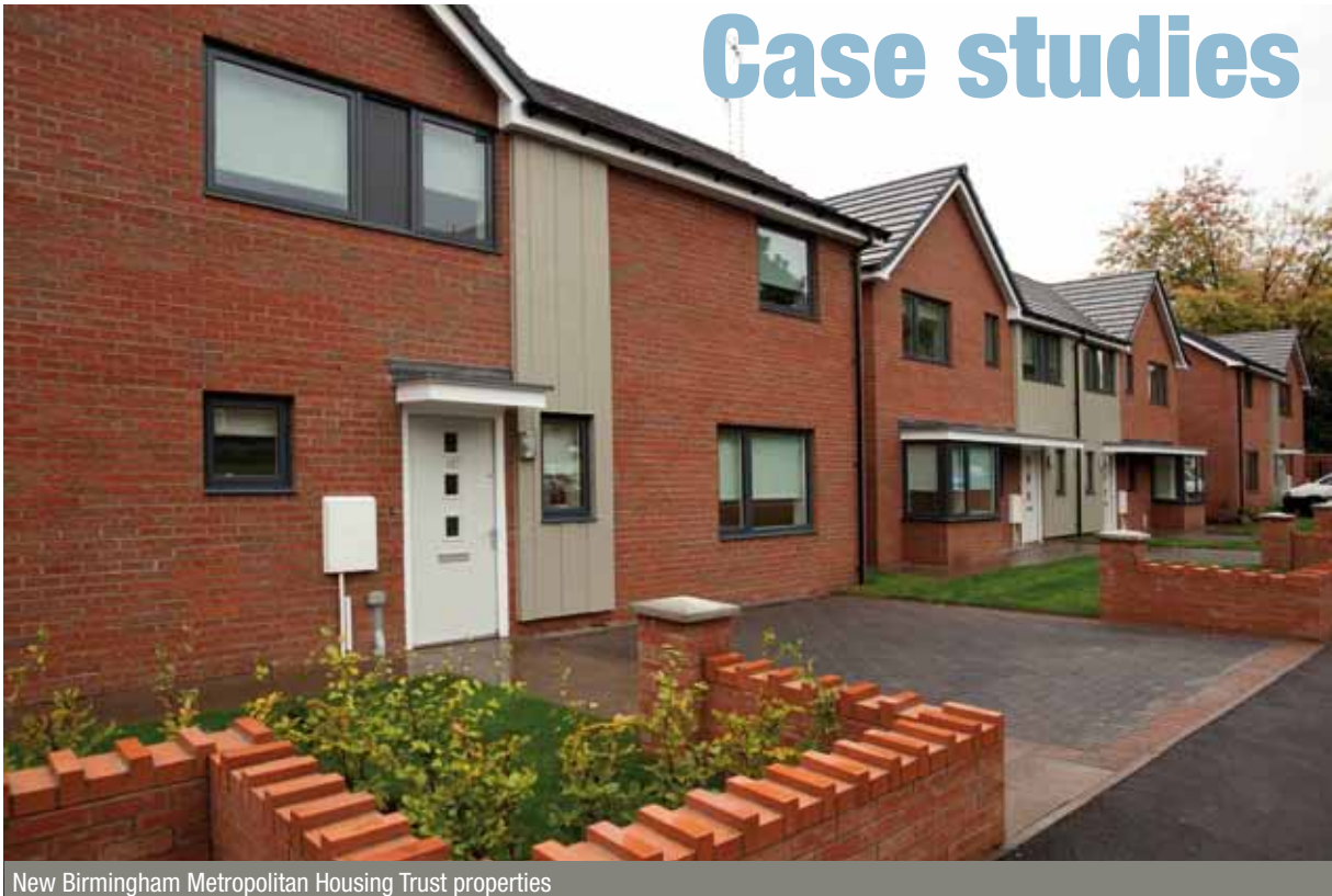
New Birmingham Metropolitan Housing Trust properties
