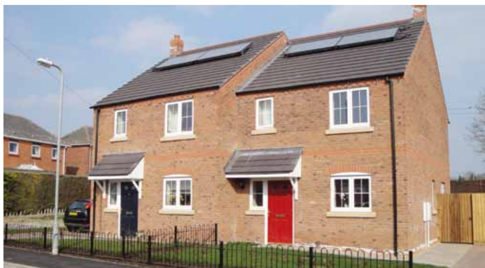
New family homes built by North Kesteven District Council
