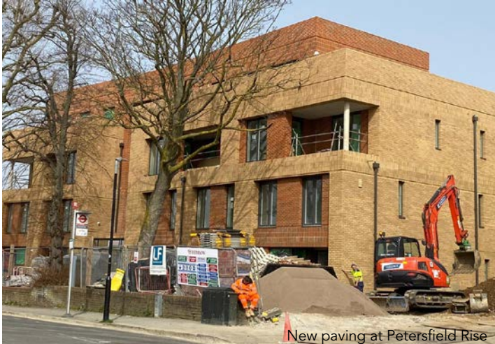
New paving at Petersfield Rise
